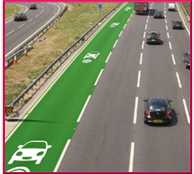
Figure 39: Wireless in road charging
